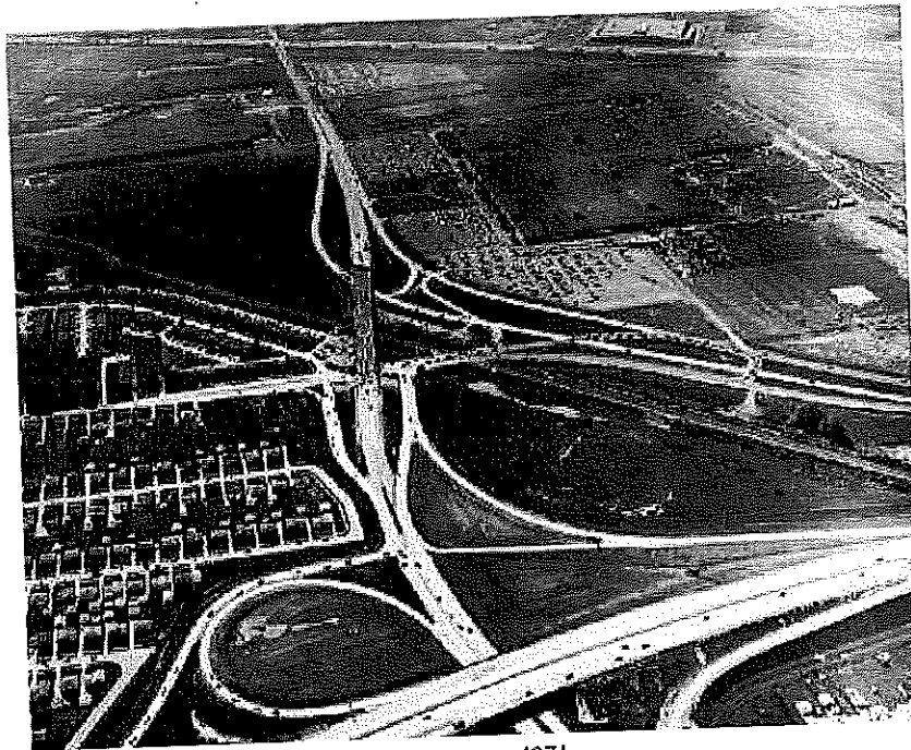
Photo: Snow Rd. Bridge I-71 to Berea Freeway, 1974.
